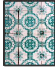
09 Tiles of English taste, produced by stamping and traceable to the Factory Louça de Sacavém (end of the 19 th century, beginning of the 20 th century).
